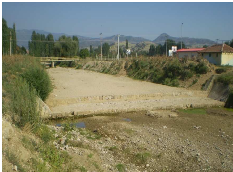
Picture No.2 Existing cascading thresholds riverbed of r.Kozjachka, village Karbinci
